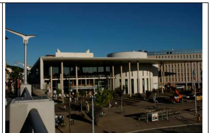
Concert Hall Freiburg, Germany
